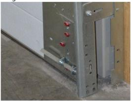
Two low headroom brackets can be installed on each side of the door to add additional reinforcement for long stem rollers when using single bottom brackets with double end stiles.
